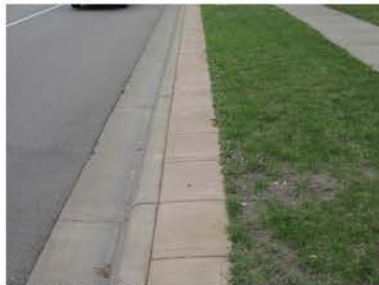
Paved Maintenance Strip
