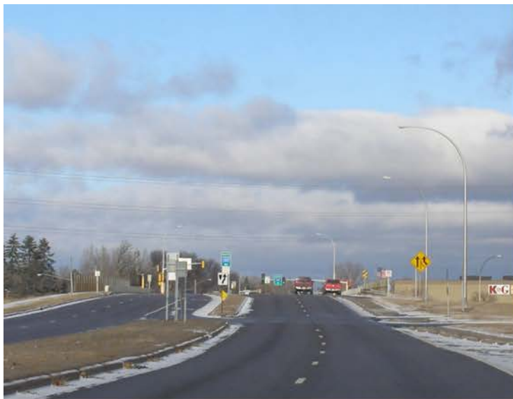
Existing Bridge Approach - Looking North
