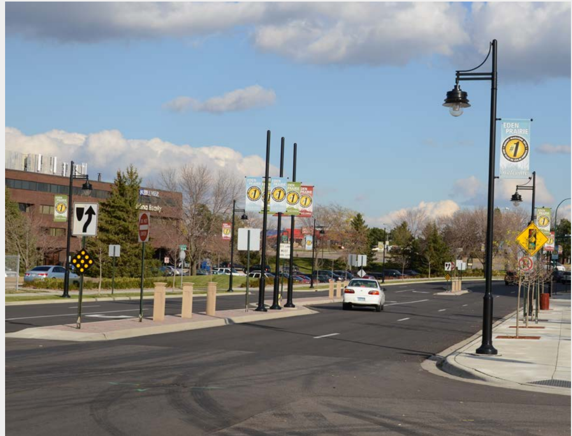
Example of median with bollards and signs – Eden Prairie
