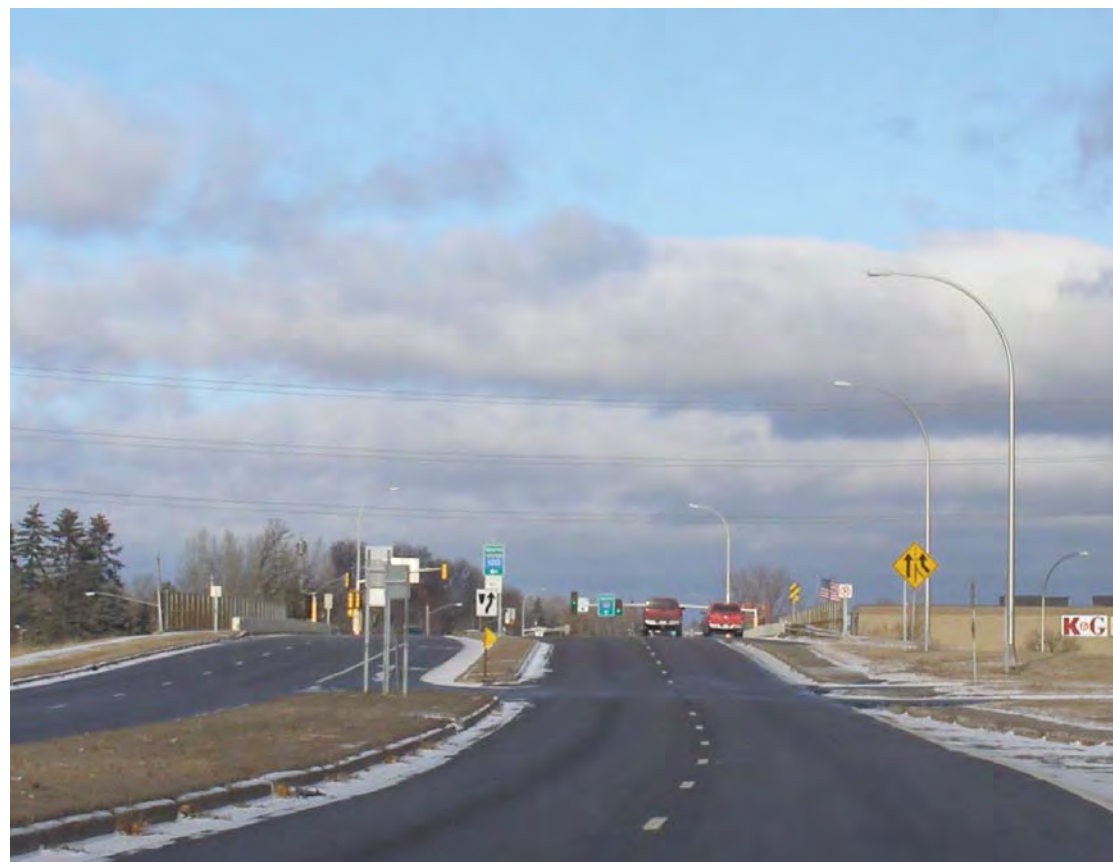
Existing Bridge Approach - Looking North
