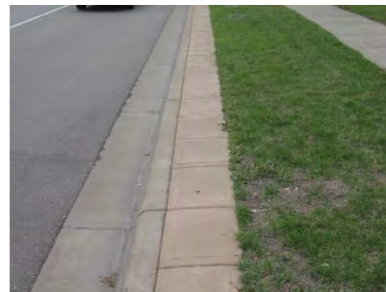
Paved Maintenance Strip
