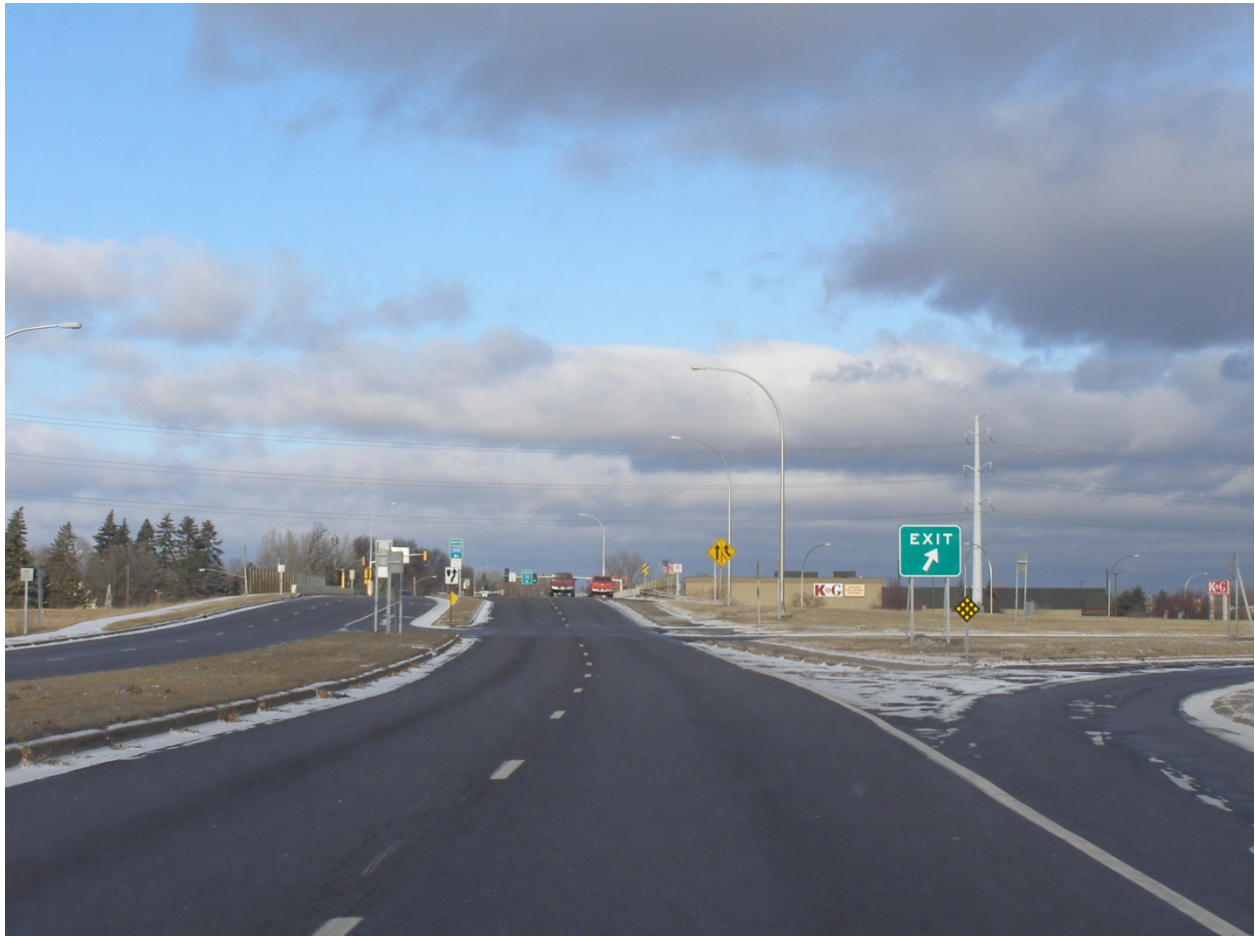
Figure A - View of Brooklyn Boulevard Looking North Approaching the TH 100 Overpass
