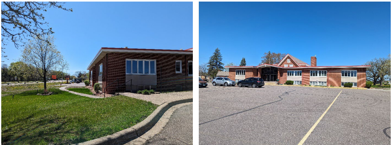
Image 1. Existing Site Conditions at Subject Property.
