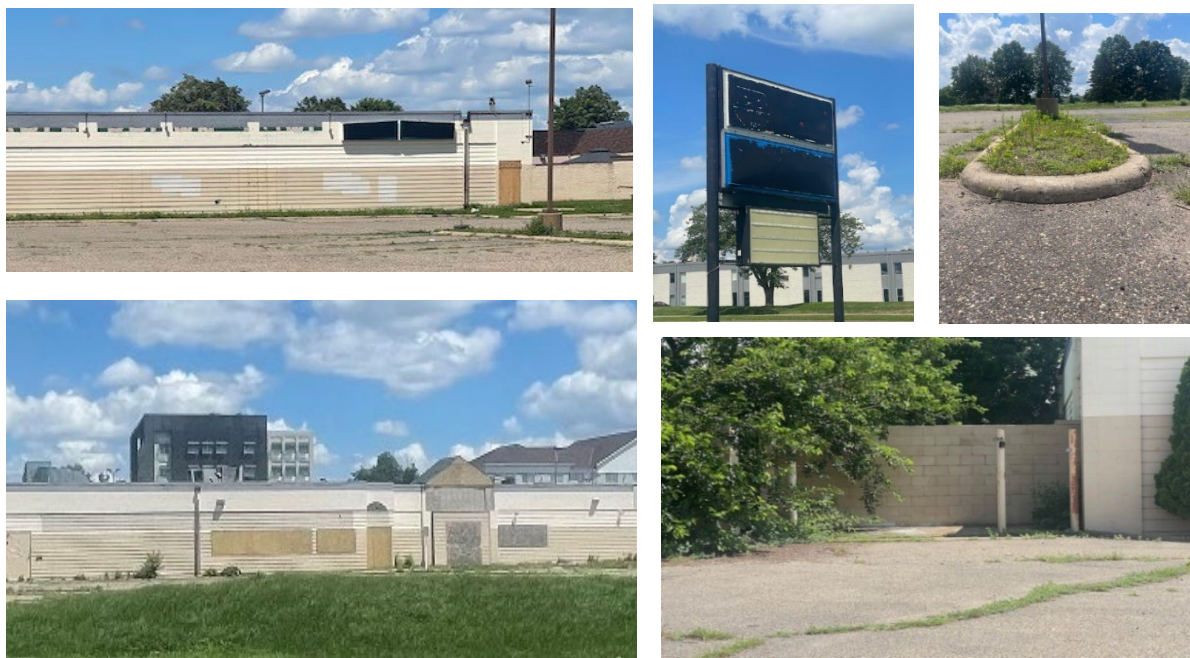
Image 1. Existing Conditions at Subject Property.
