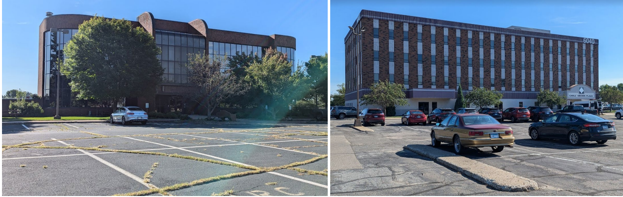
Image 2. Existing Parking Conditions at Different MX-B District Properties.
