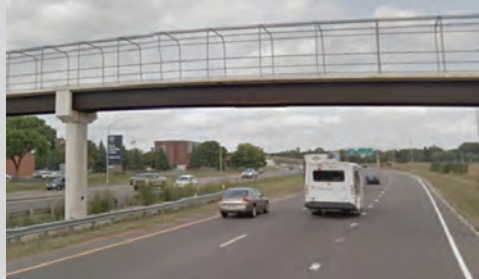
Pedestrian Bridge over Hwy 100
