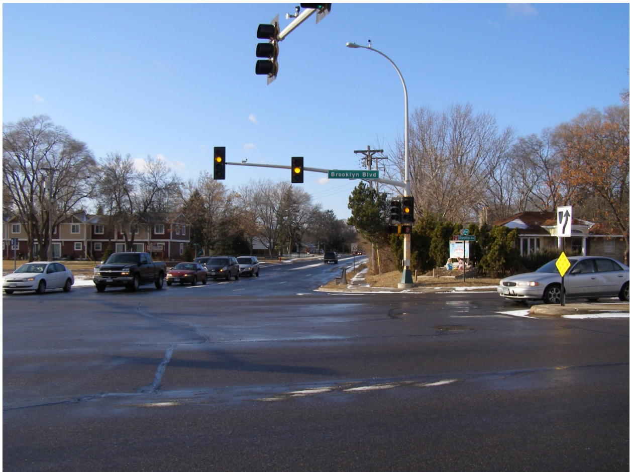
Figure B - Existing 63rd Avenue Intersection Crossing at Brooklyn Boulevard
