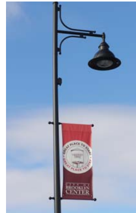
Intersection/Boulevard Lighting With Banners
