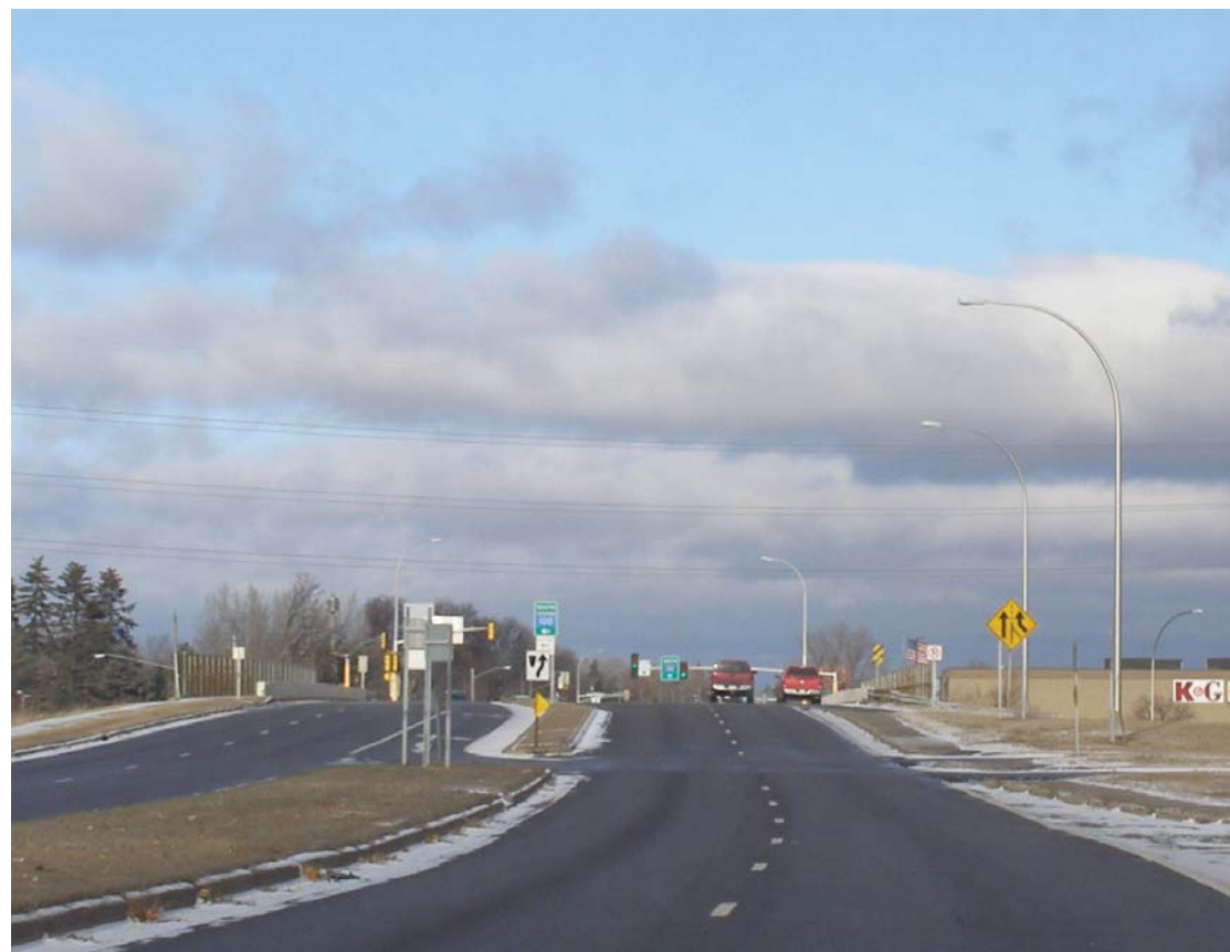
Existing Bridge Approach - Looking North
