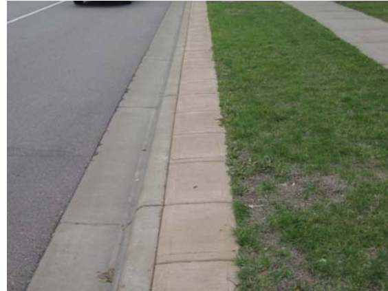
Paved Maintenance Strip
