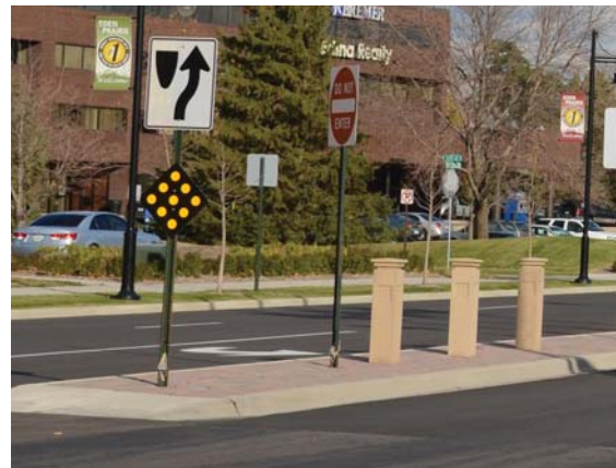
Paved Median (includes bollards, colored paving)
